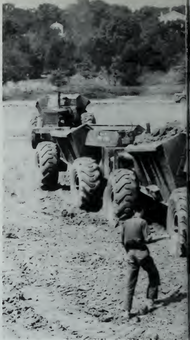
Preparing the site, Arlington Cemetery in background
